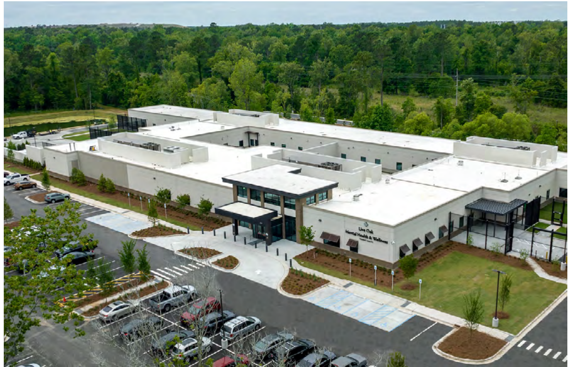
HCA Live Oak Mental Health & Wellness, completed by HKS Architects.
