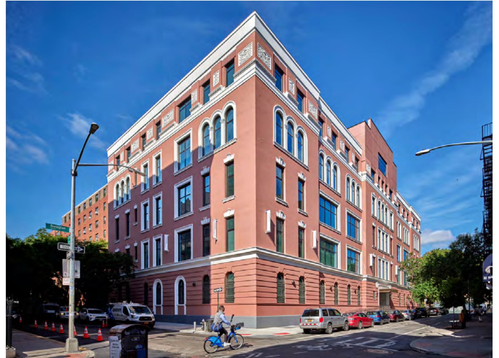
Images of the Mount Sinai Beth Israel Comprehensive Behavioral Health Center renovation project. Created by HKS Architects.
